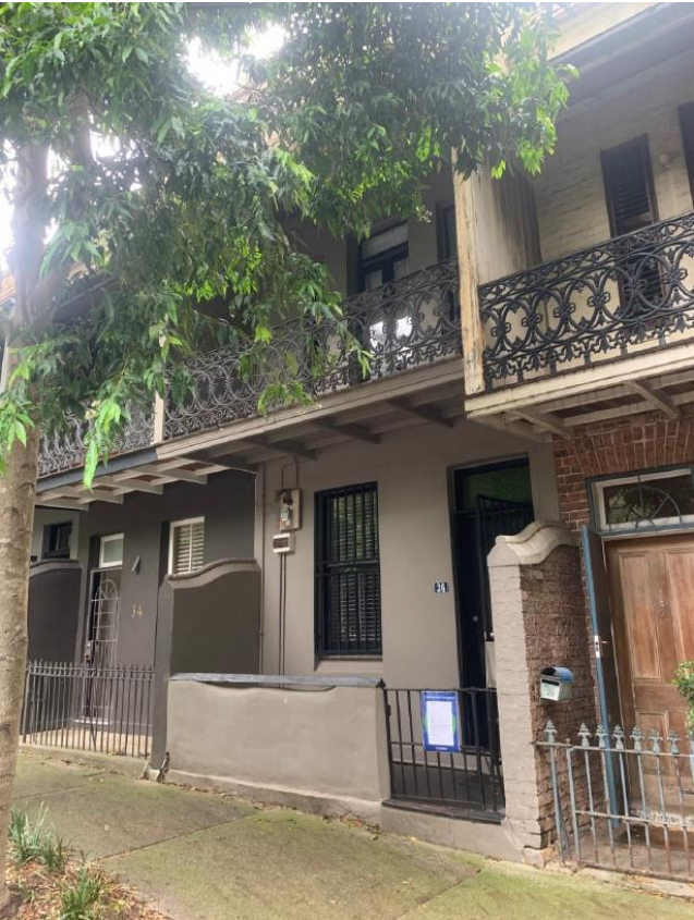
Figure 4: View of the site from Selwyn Street
