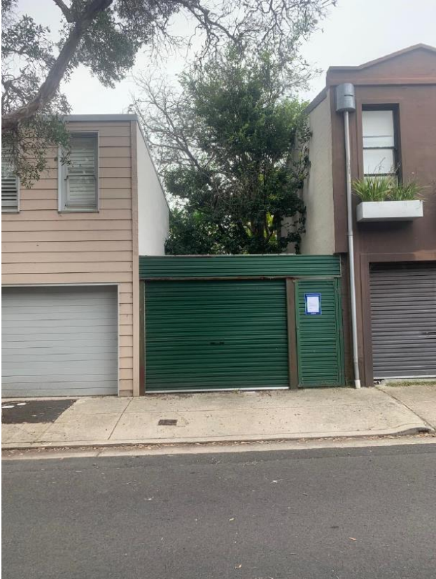
Figure 2: Site viewed from Iris Street
